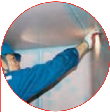
Inspection of stripe coats.
