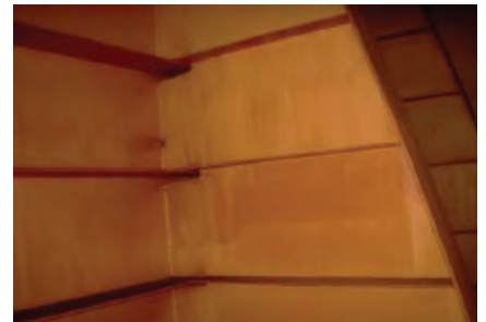
Chemical carrier after 3.5 years in-service
